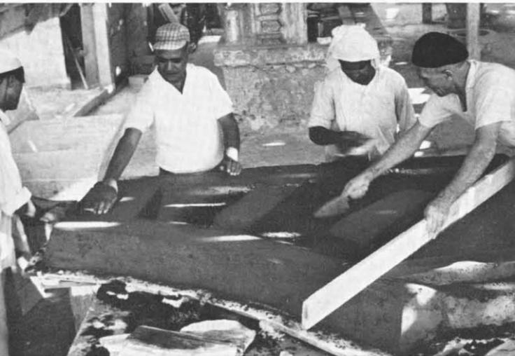
No marble is wasted. Residue from cutting and finishing operations is crushed, mixed with binder, then poured into mold to make cast marble. At right, craftsmen inspect finished panel after removal from mold.
