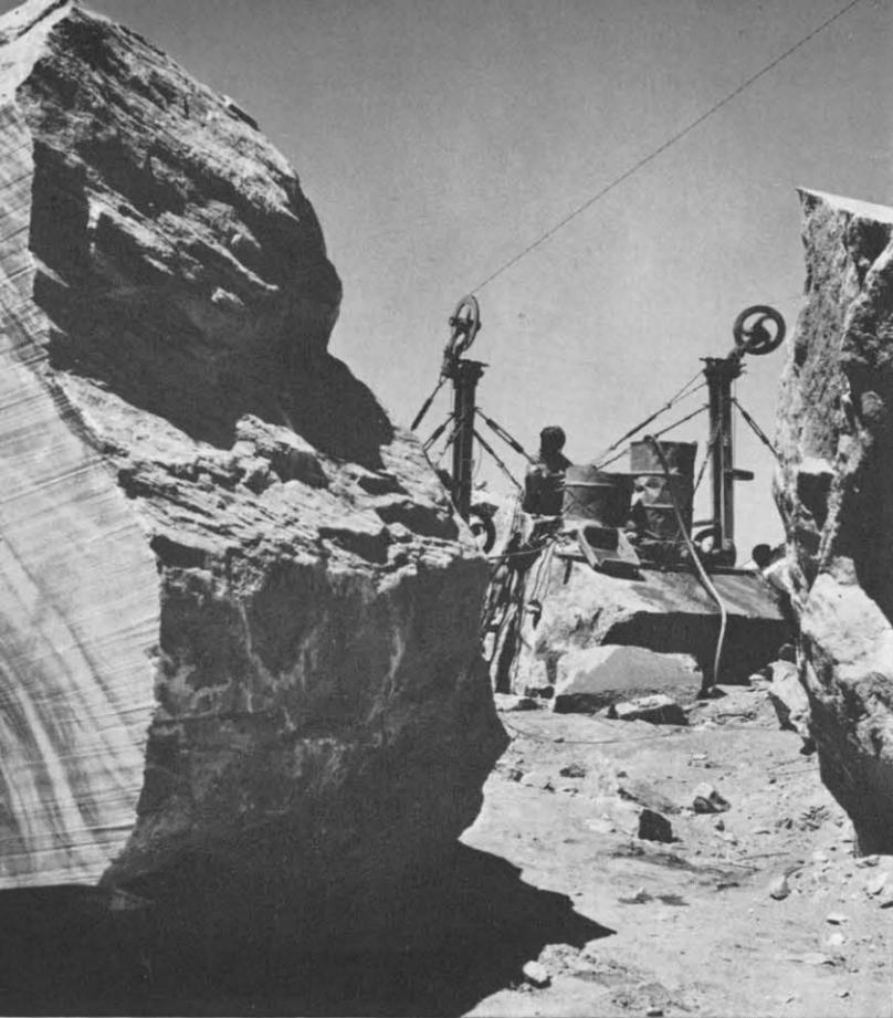
Blast-loosened marble boulders are rough-cut at quarry by wire ropes, giving flat surface seen at left of boulder. Wires, aided by water and sand, cut at a rate of two to three feet a day.
